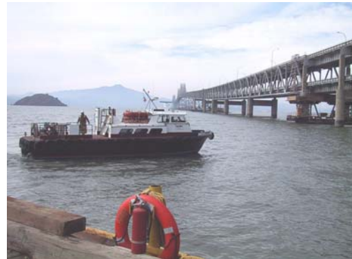
View of the Richmond San Rafael Bridge.
