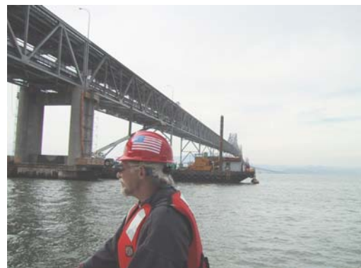
Bridge with view of Drill Platform and Barges
