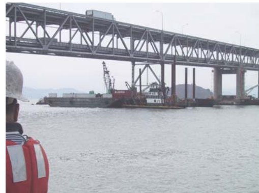
Drill platform with drill rig.
