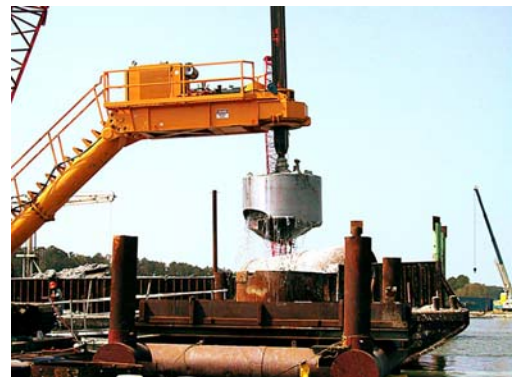
Crane Mounted drilling attachment allows deeper holes to be drilled.(click image to enlarge)
