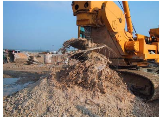
View of spoils spinning from auger. The polymer can be seen flying off the auger. Notice how dry the spoils stay.
